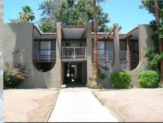
97 UNIT UNDER $42,000 PER DOOR Mesa
